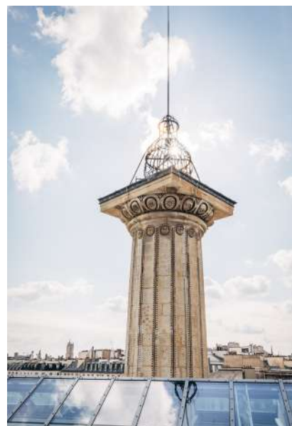
Photo Vladimir Partalo, mars 2020. © Bouygues Construction.
